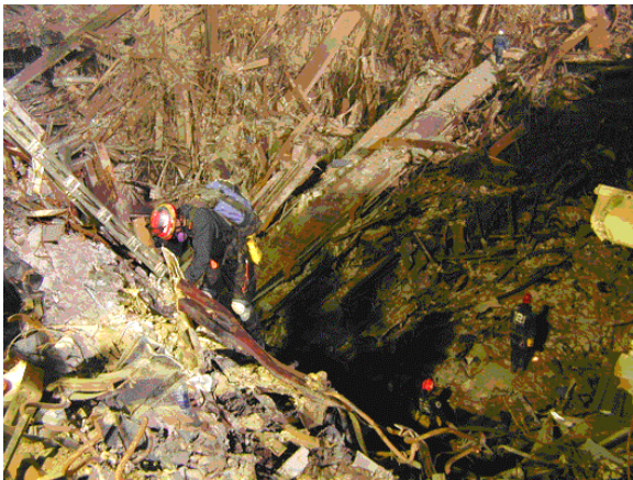
Figure 9-3 - GZ workers descend into the subbasements below WTC2. While there is extensive damage, there is little building debris at the bottom of the hole. There is no
