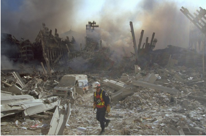
Figure 9-6 here again we see the "rubble pile" from WTC1 is essentially non-existent. The ambulance is parked at ground level in front of WTC1. WTC6, which had been an eight-story building, towers over the remains of WTC1.
